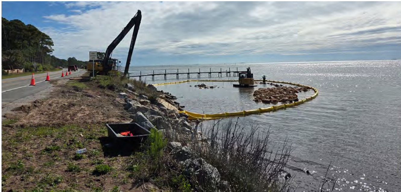
Fresh limestone rocks in a completed Phase 2 reef, with further construction occurring in the background on 4.14.26.
