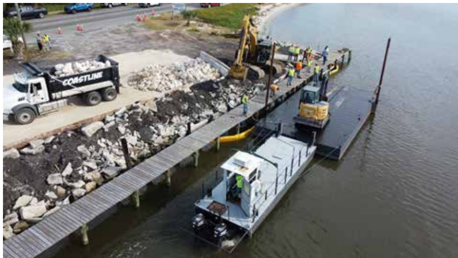
Limestone materials for the project site are loaded onto the barge in the image above.
