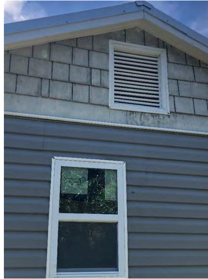
Figure 3: Vinyl siding and new windows were added; another effort to reduce energy bills and protect the overall envelope of the home.
